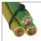
Nylon cable tie tensioned and cut i.e no sharp edges
